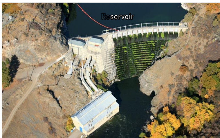
Figure 4.2-7: Photo of Copco 1 Dam and Reservoir with specific components labeled. With full facilities removal, all visible components would be removed. With partial facilities removal, certain components (e.g., penstock) would be retained.
